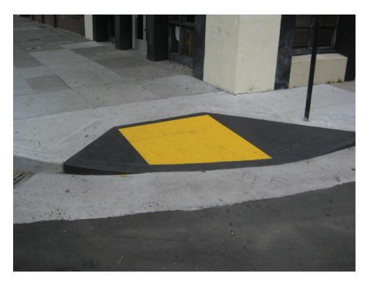
Figure 5: Example ADA-compliant curb ramp
