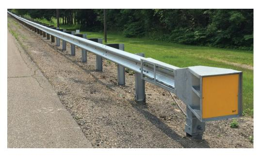
Figure 3: Example Midwest Guardrail System with crash cushion
