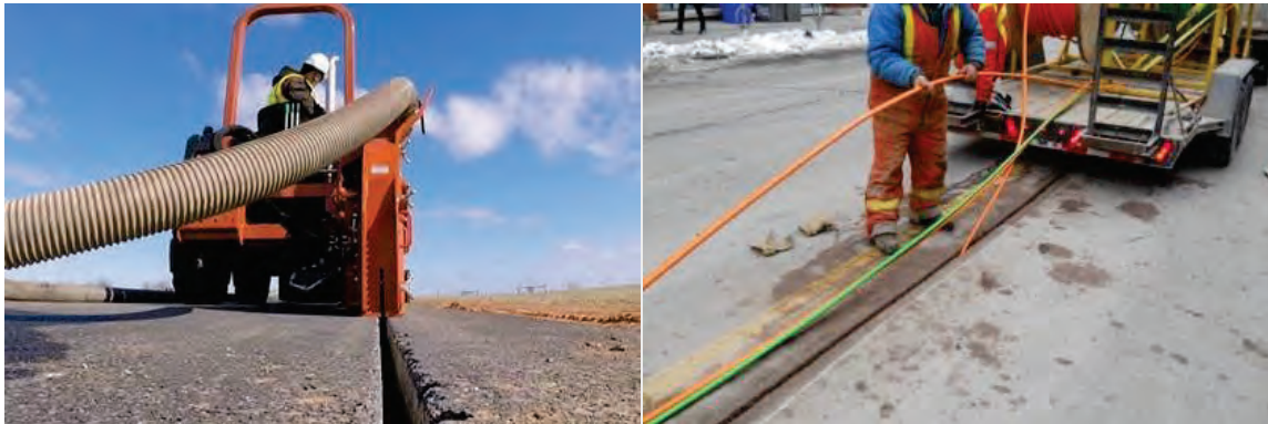
Figure 2-7 Trench in Pavement Method
