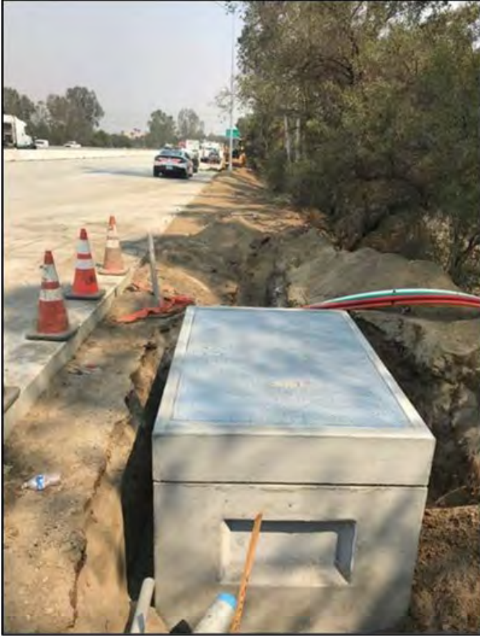
Figure 4. Vault Installation Maintenance Vehicle Pullouts
