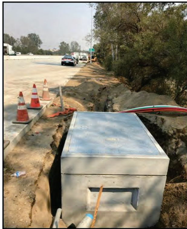
Figure 2-2 Pull Vault Installation
