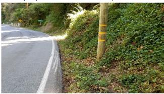
Photos 4 & 5 Loma Mar Section-Top photo 4: some recovery area on approach to curve, shoulder widening. Bottom photo 5: fixed object, no allweather shoulder, edge drop-off. Photo credit: FHWA
