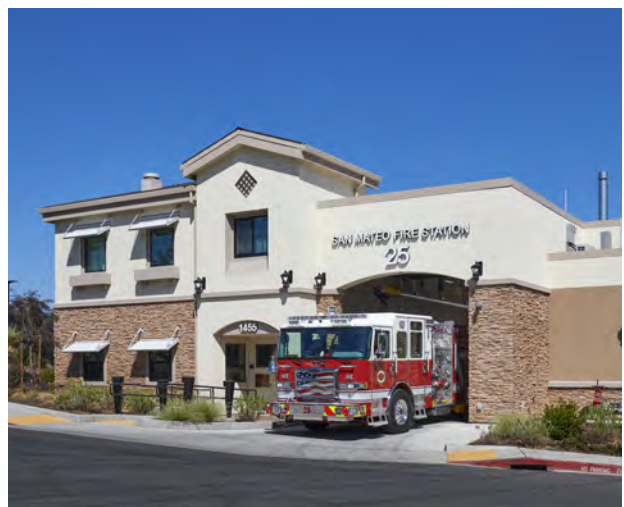
San Mateo Fire Station 25
