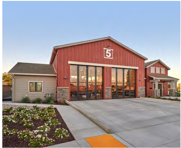
Manteca Fire Station 5
