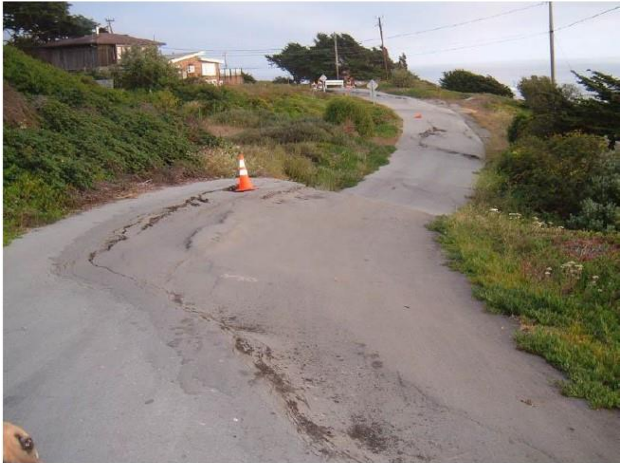
Picture 10: Slip on active scarp visible as slip line cracks in the road, as is a fault line settlement as the large dip in the road.
