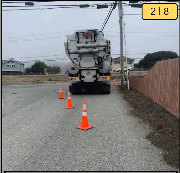
Set up cones and signs as necessary to keep the public out of your work zone.
