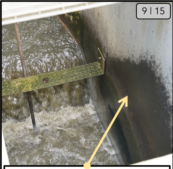
Spray down the channel walls of all scum & debris.
