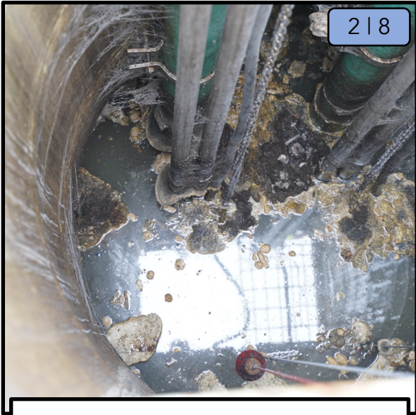
Visually inspect the well for grease and debris.
