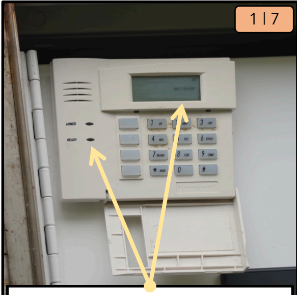
Check that all alarms are off. The code should show "Ready" with the green light illuminated.
