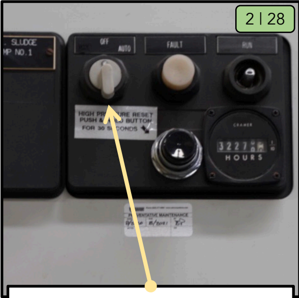
Turn the HOA switch to the "Off" position.
