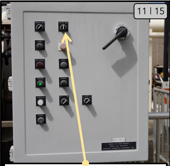
While in HAND, use the forward/reverse switch to move the conveyor to the optimal position for cleaning each of the following parts of the bar screens.
