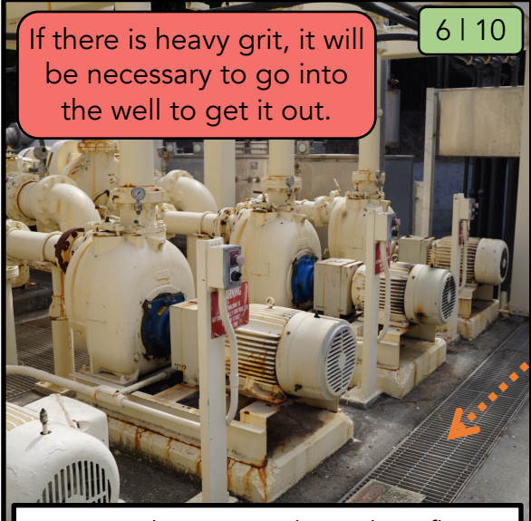
Remove the grating above the Influent Wet Well. Then, using the hose wash the grit into the pump suction lines a little at a time.
