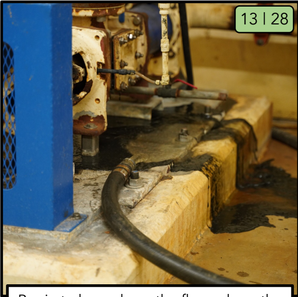
Begin to hose down the floor where the sludge discharges from the pump to ensure it is flowing toward the channel and drain.
