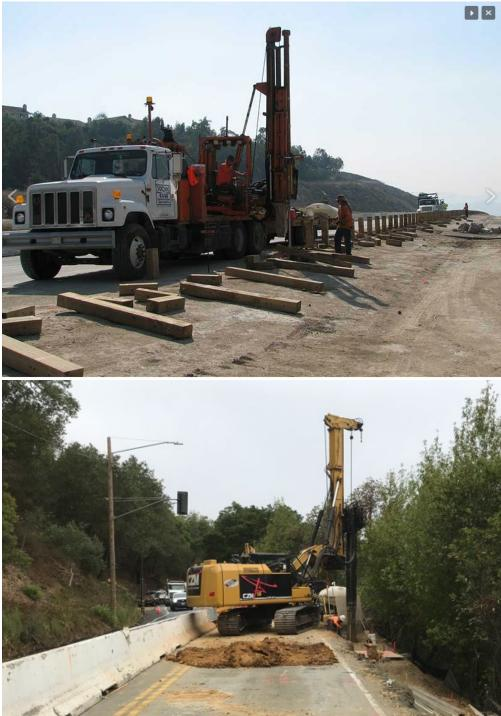
Figure 1-6 Examples of Barrier Installations (Page 1 of 2)
