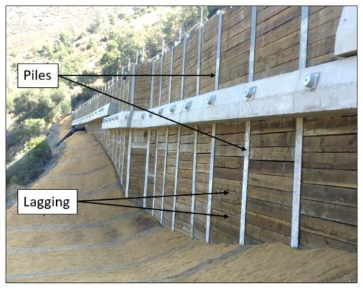
Figure 1-5 Example Soldier Pile Retaining Wall
