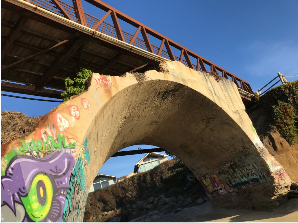
Arch bridge looking at the west side of bridge – January 2021
