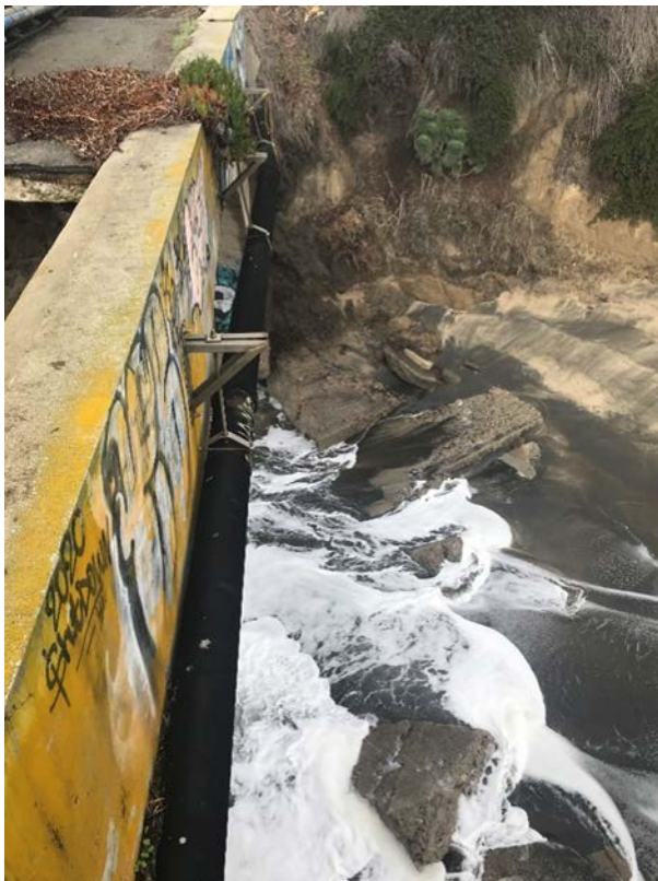
Abandoned sanitary sewer pipe on the east side of bridge
