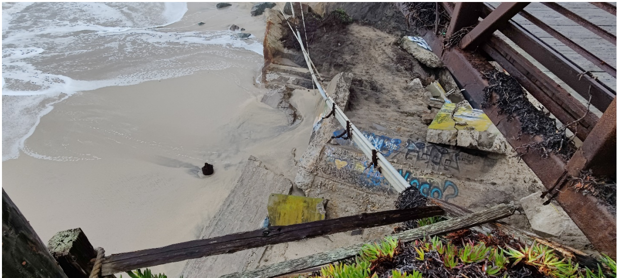
Mirada Road Bridge after 12/15/2021, west side of bridge.
