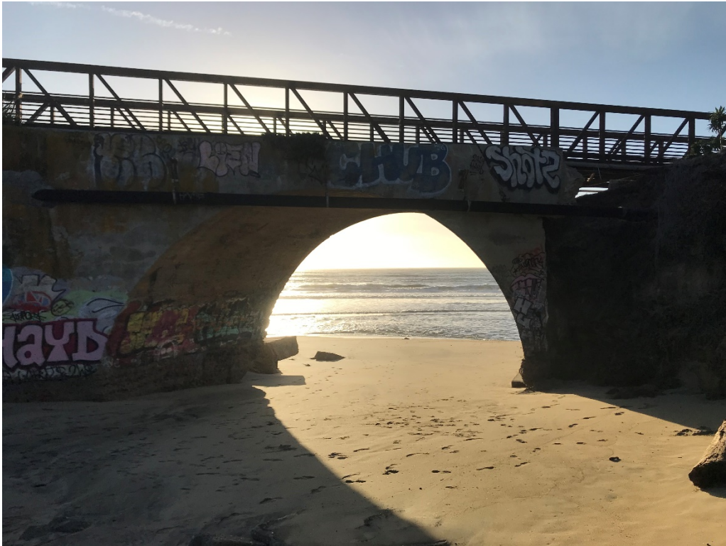
Arch bridge east side looking towards the west – January 2021
