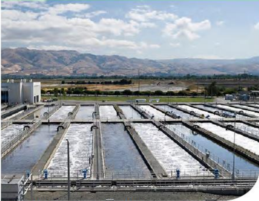
Eastward view of secondary treatment tanks
