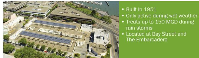
North Point Wet Weather Facility
