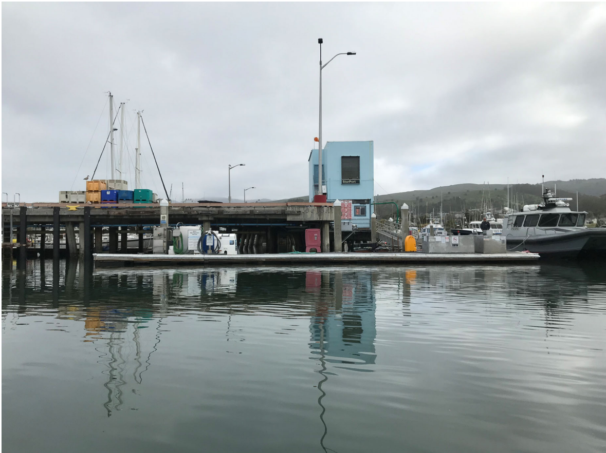
71 – View of Fuel Dock from water
