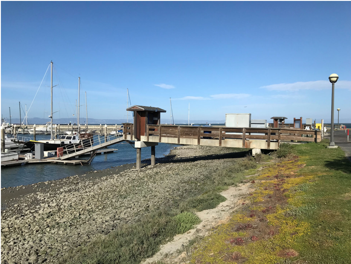
38 – View of East Basin Dock 13 gangway platform
