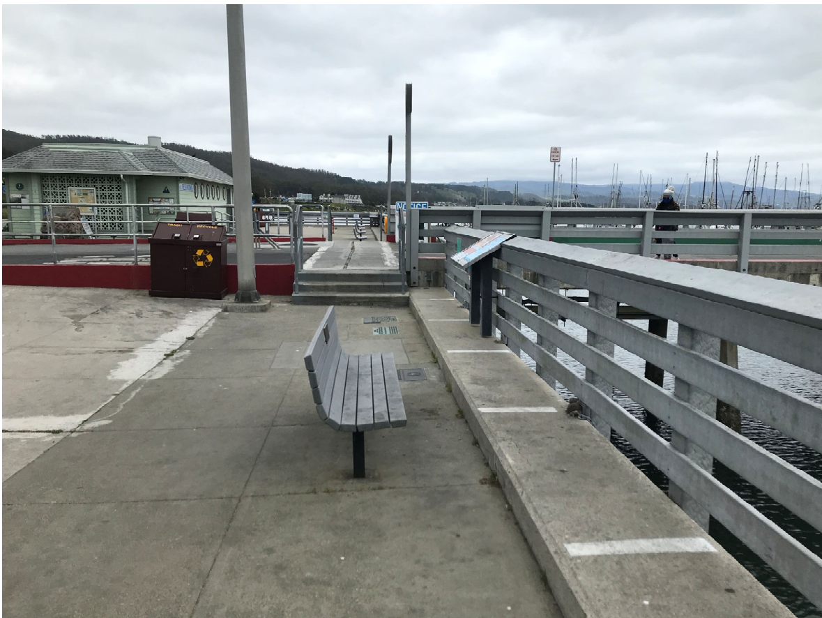
17 – View of promenade at base of pier
