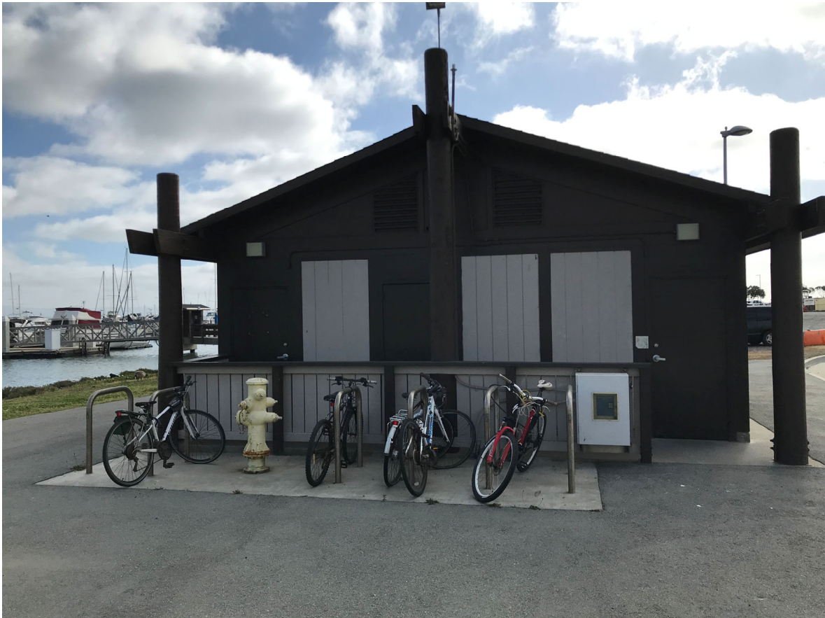
61 – View of East Basin Restroom 3
