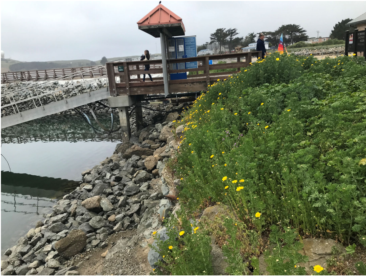
22 – View of rock slope and Docks A-C gangway platform
