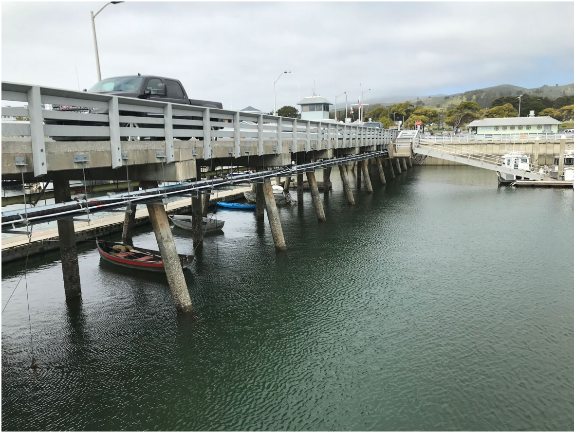
2 – View of east side of Johnson Pier
