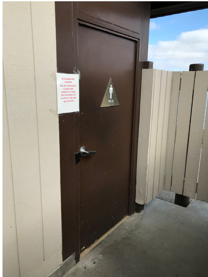
63 – View of East Basin Restroom 3 exterior door and paint
