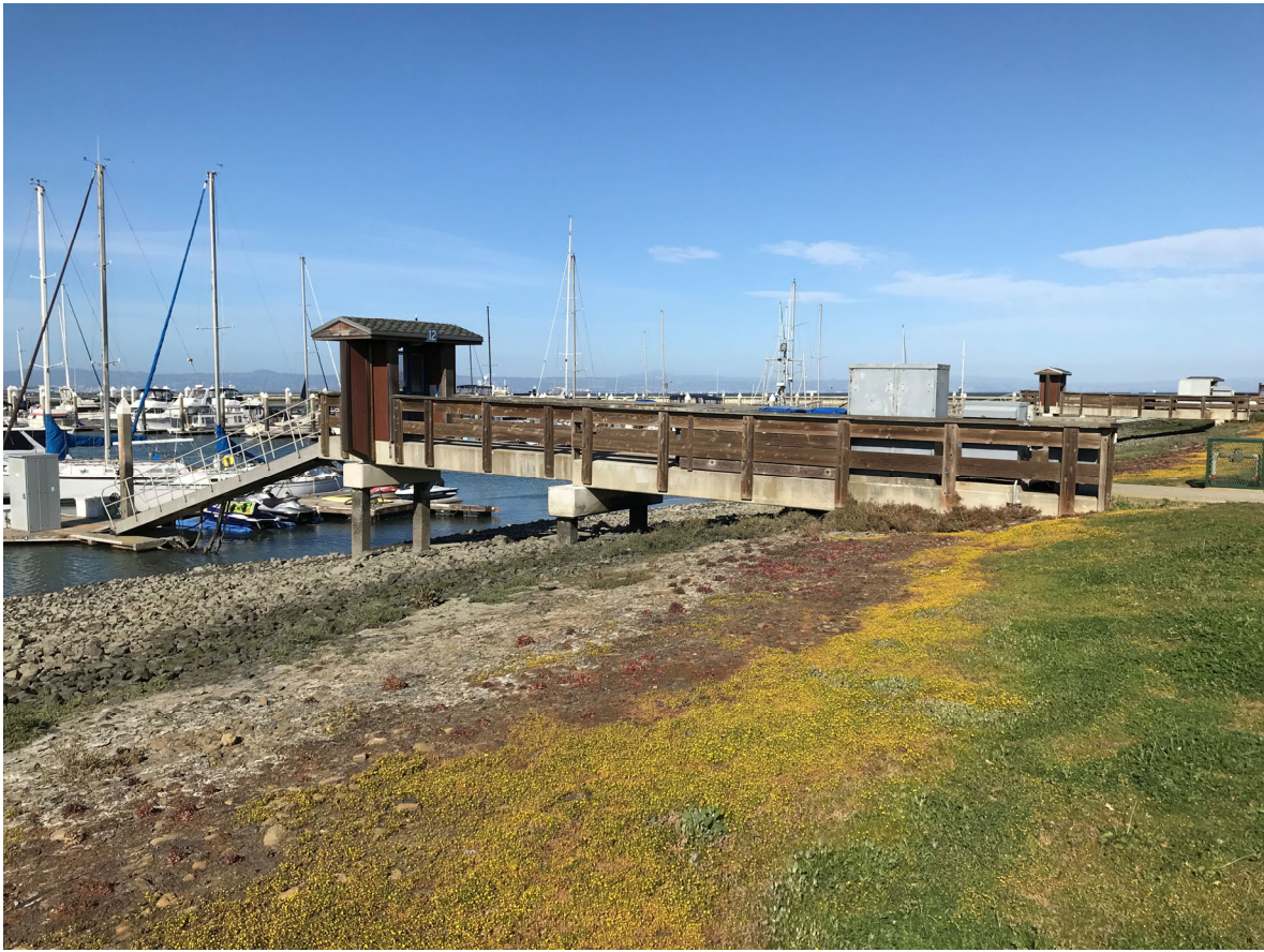
32 – View of Dock 12 gangway platform
