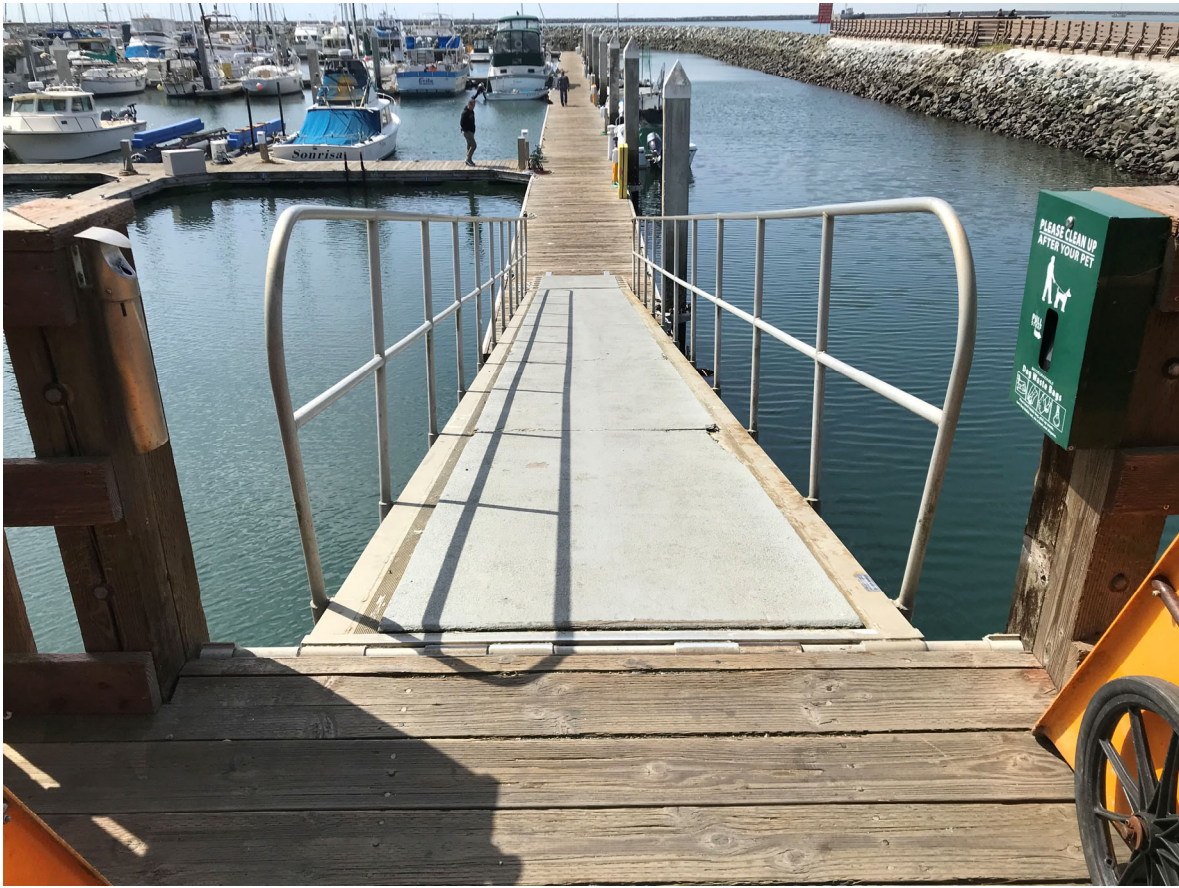
50 – View of Dock A-C gangway and main walkway
