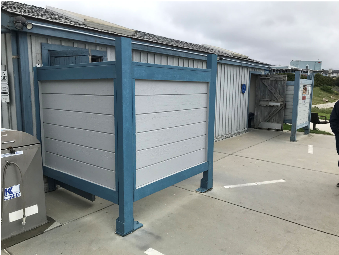
44 – View of East Restroom with new men's privacy screen
