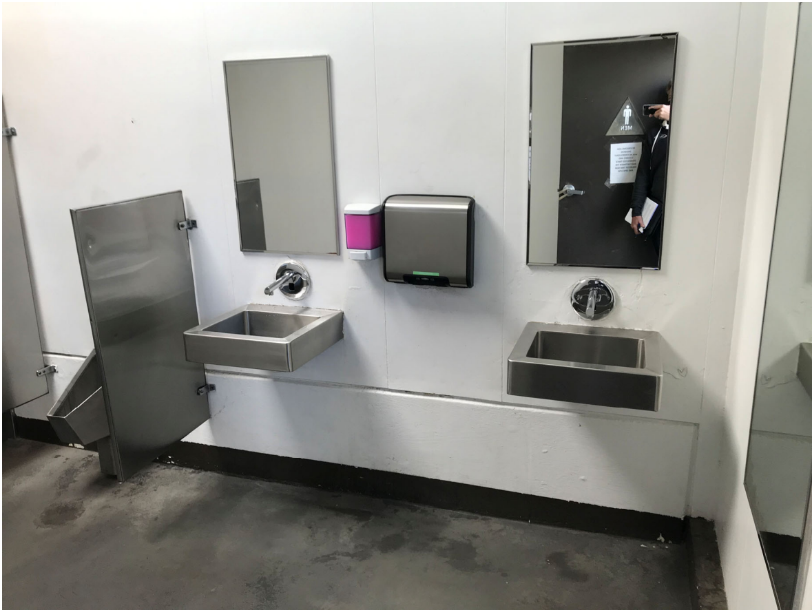
56 – View of Restroom Building 1 interior
