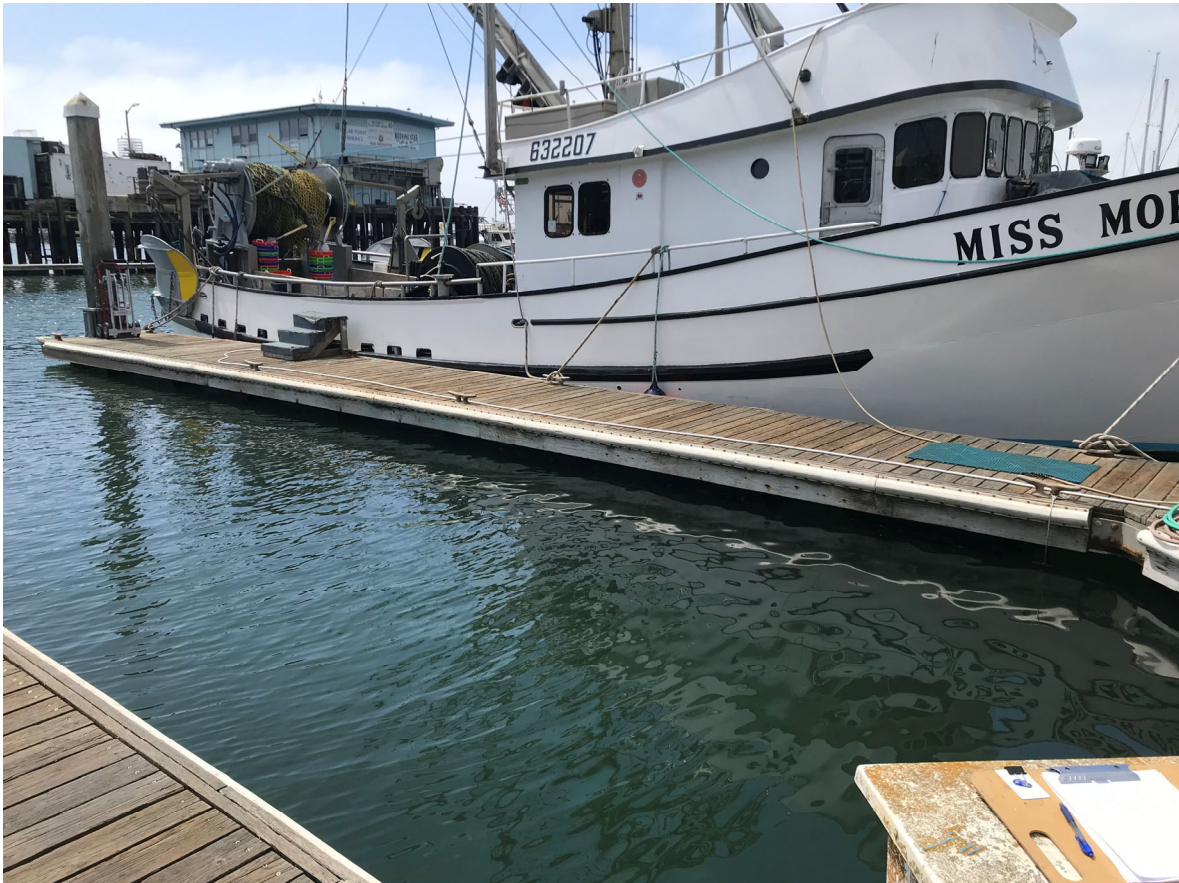
61 – View of typical Dock E finger
