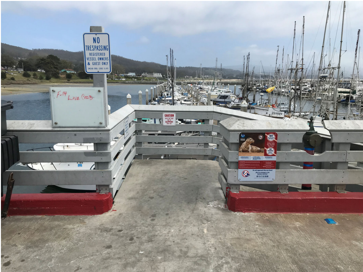
63 – View of entrance to Dock F
