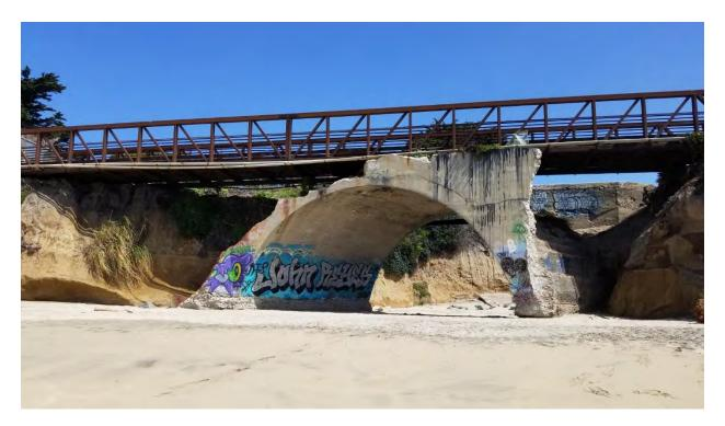
**Figure 3.** Cement arch bridge supporting current pedestrian bridge.
