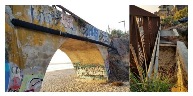
**Figure 7.** Existing infrastructure (sewer main and PG&E electrical conduit) located on pedestrian bridge and cement arch bridge.
