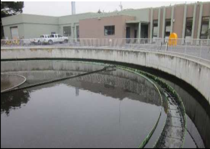
Clarifier: separating out water for treatment
