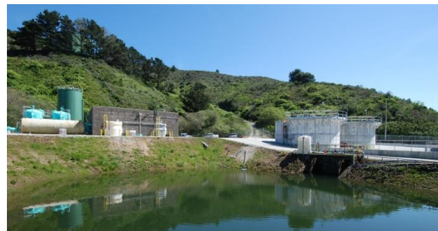
Denniston Water Treatment Plant
