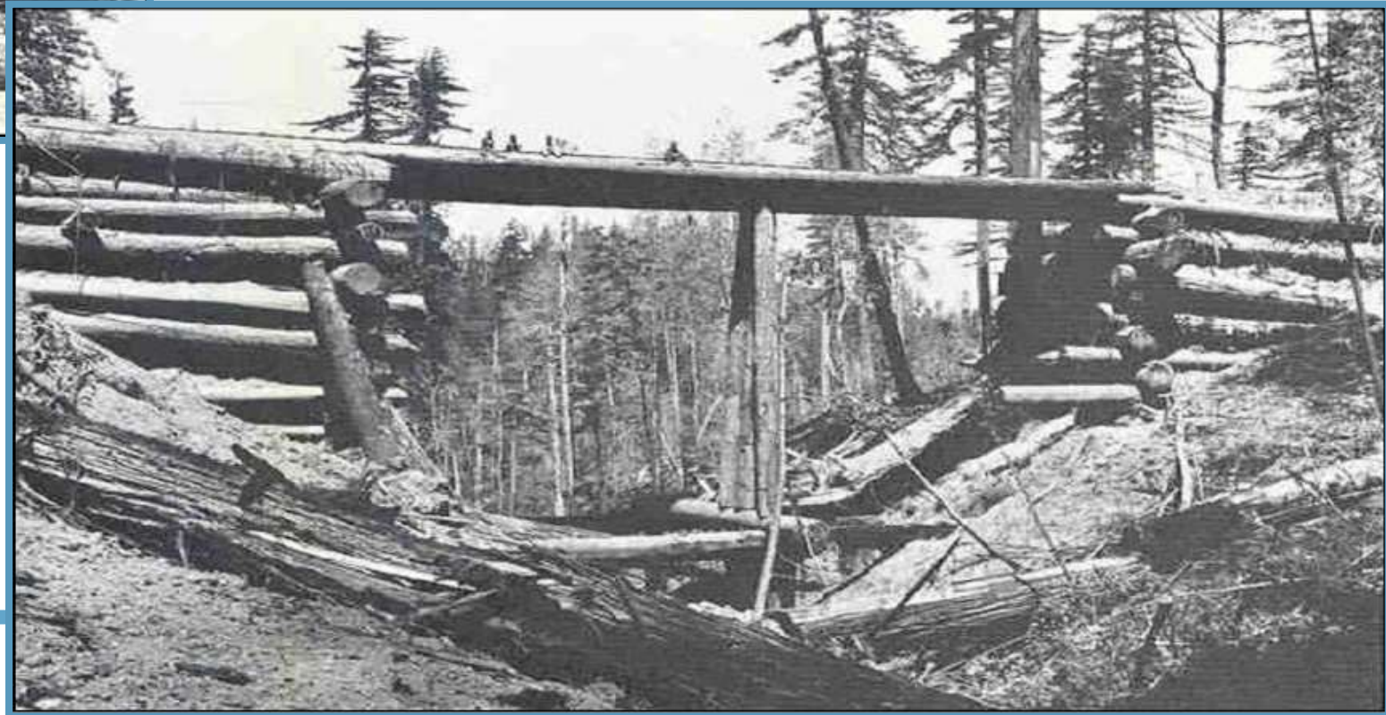
Crib log, or "Humboldt," creek crossing on Old Haul Road. Note men sitting on top of the crossing. Photo: Santa Cruz Lumber Company (1943)
