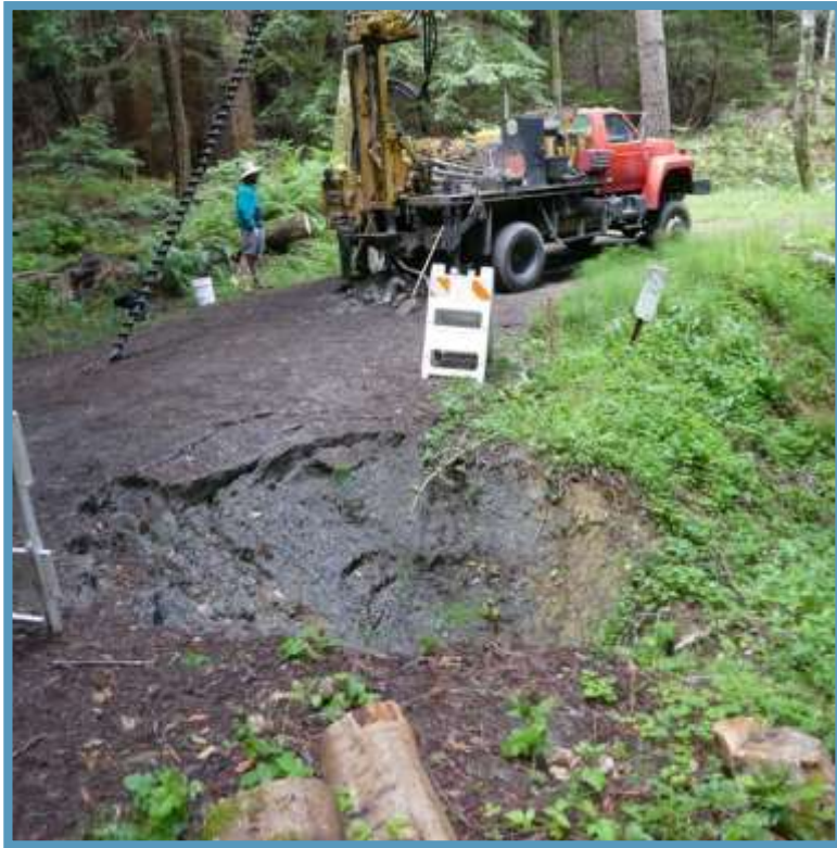
Pre construction: Harwood Creek crossing (2017)
