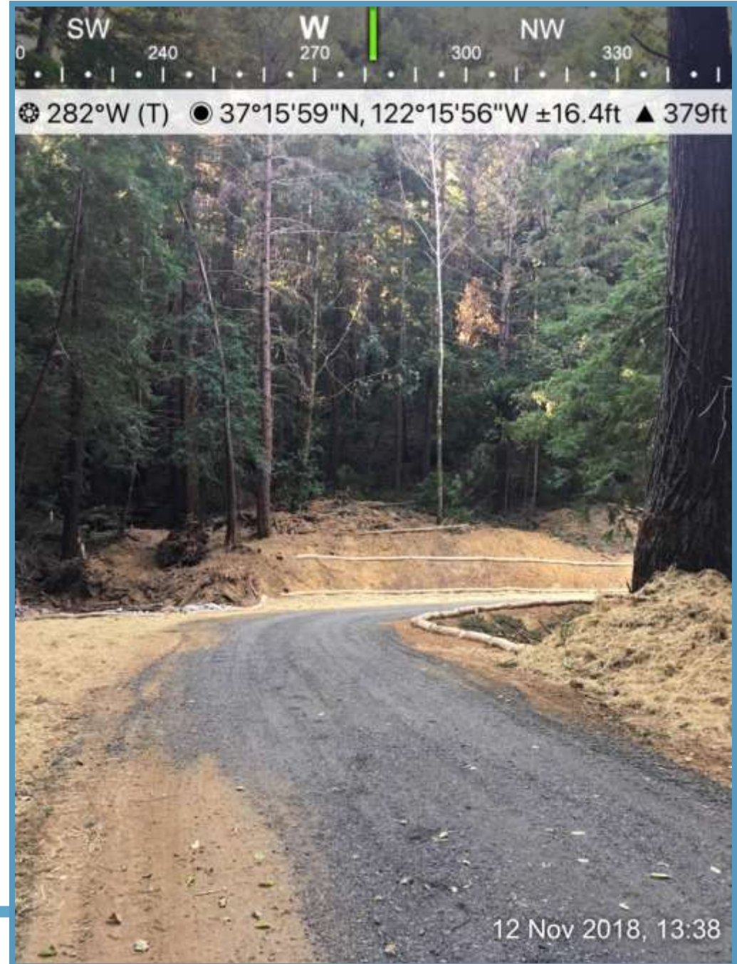
Post construction: Harwood Creek crossing (Nov. 2018)
