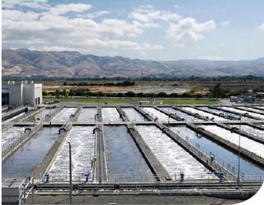
Eastward view of secondary treatment tanks
