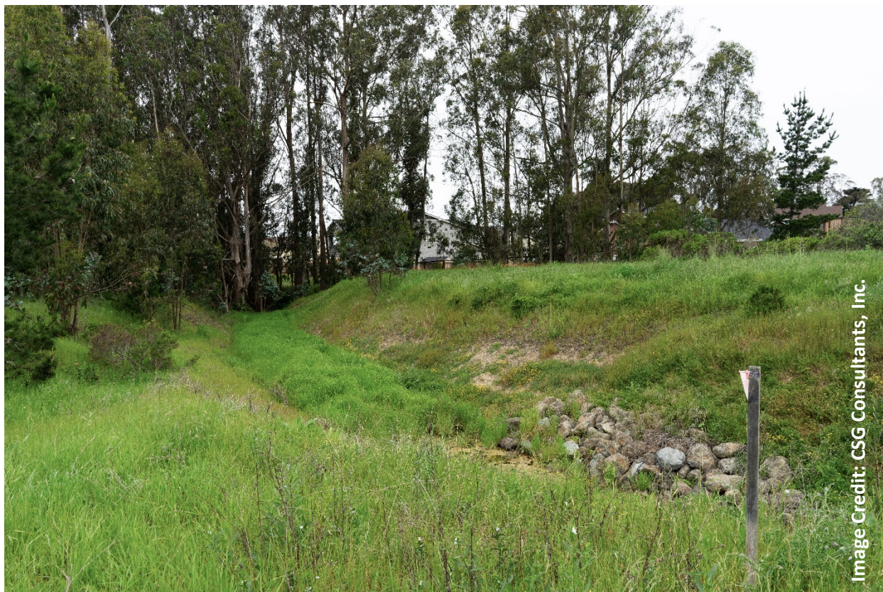
Bioretention swale located at Pacific Ridge Subdivision.
