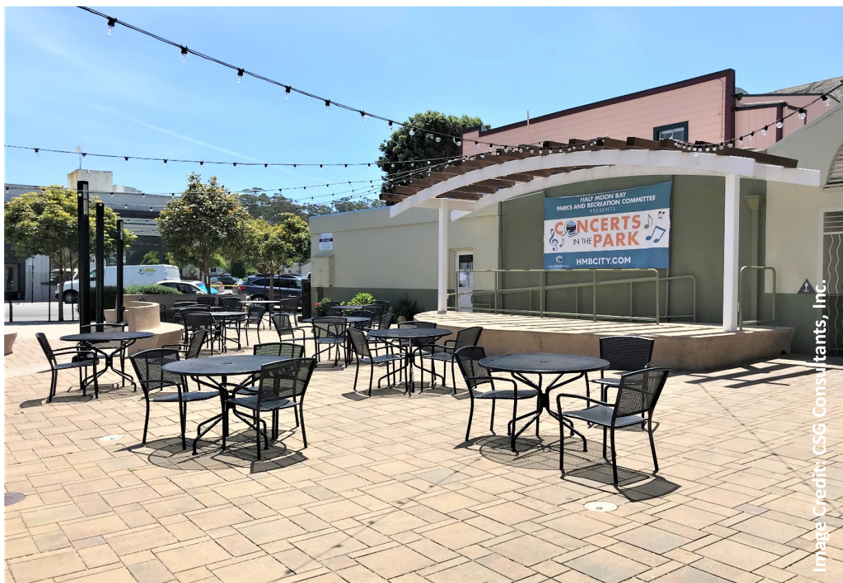
Permeable pavers located at Mac Dutra Plaza.
