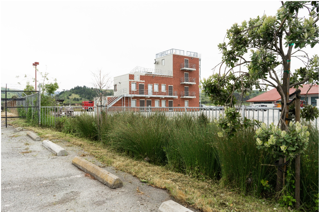
Bioretention area located at the fire department training lot.
