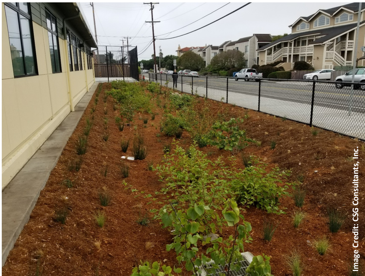
Bioretention area located at Hatch Elementary School.
