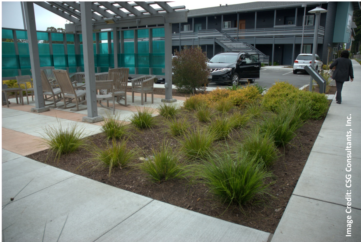
Vegetated area at the Coastside Senior Housing which receives stormwater runoff from adjacent sidewalk areas.
