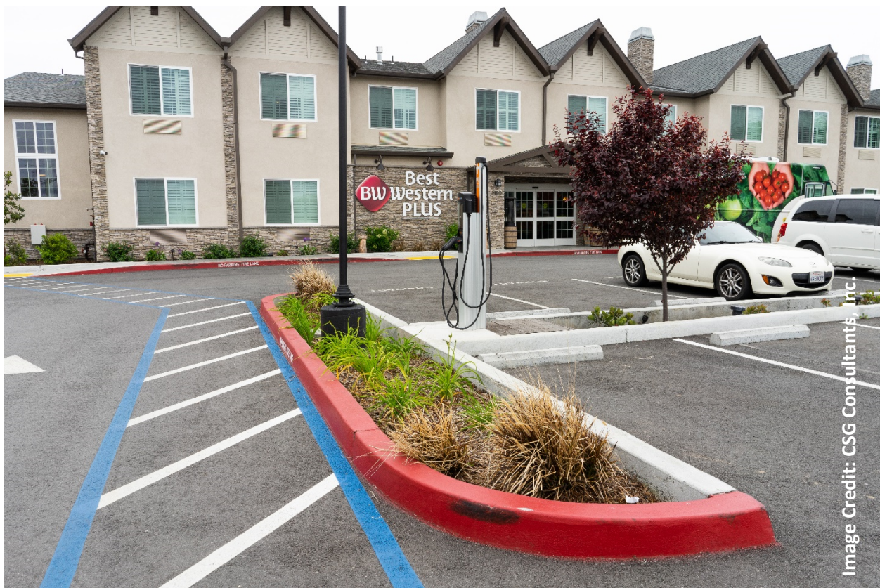
Bioretention area located at Cameron's Best Western.
